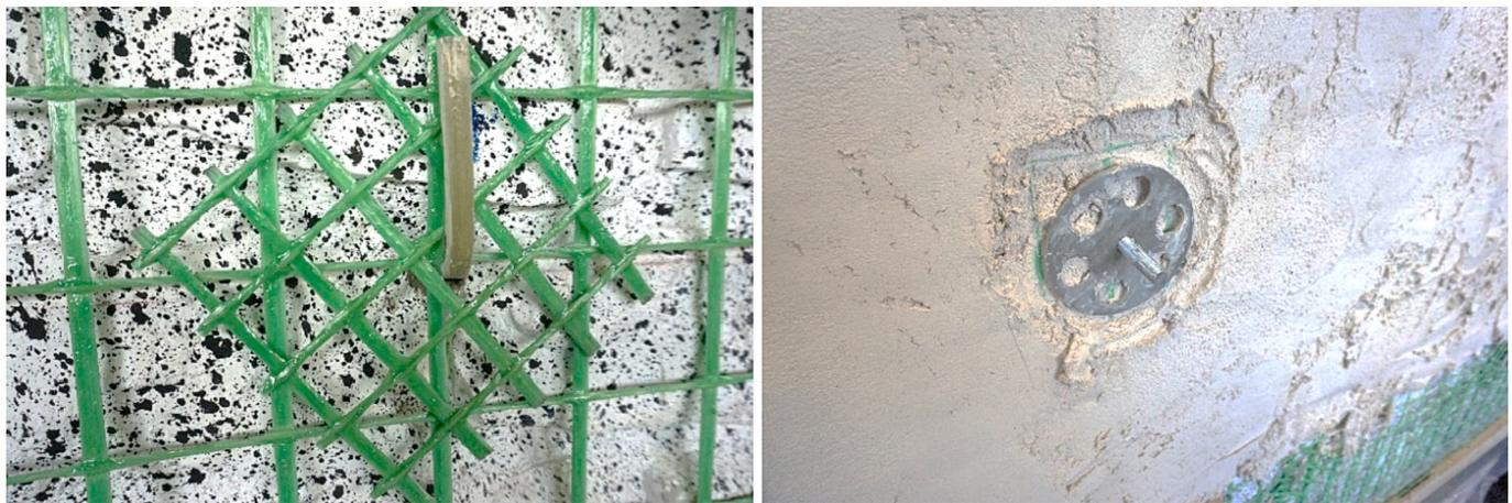
Fig. 2. View of the connectors during construction: (a) L-shaped GFRP connectors before application of coating and (b) artificial diatone during application of coating.
